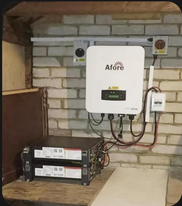
Country: UK Product: Single Phase Hybrid Inverter 6kW Battery: 8kW·h
