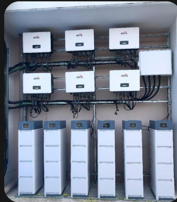
Country: Japan Product: Three Phase Hybrid Inverter 9.9kW Battery: 85.2kW·h
