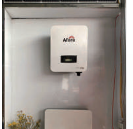
9.9kW Battery: 85.2kW-h 59.4kW Japan
